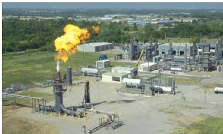
▲ **Figure 6.** This facility can test flares at the high flowrates experienced during actual plant operations.
